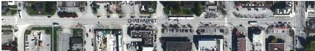
Aerial View of Chatham Street
