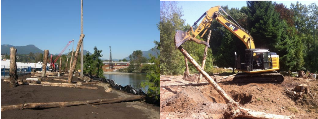
Photo 15-2: Examples of Standing Wildlife Tree Placement on Restoration Sites at Lynn Creek and in Tynehead Regional Park
