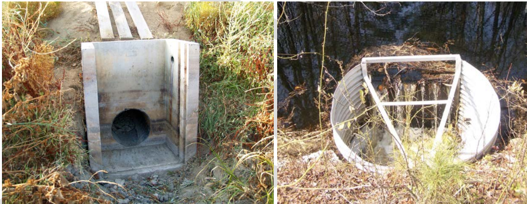
Figure 10-4: Examples of the Wetland Outlet Structures
