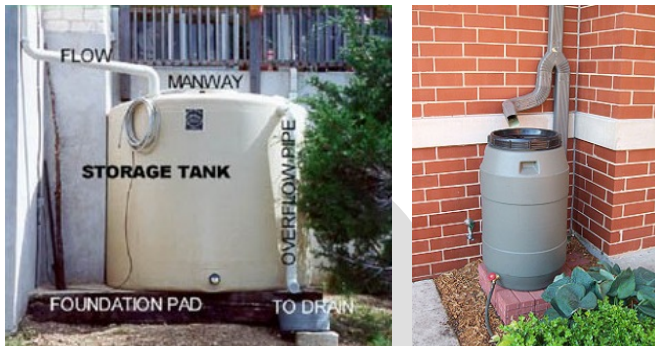
Figure 12-1: Example of Rain Barrel and Cistern
