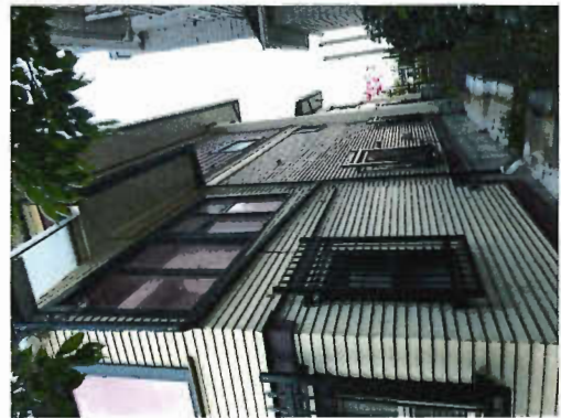
② EXISTING NORTHWEST CORNER
