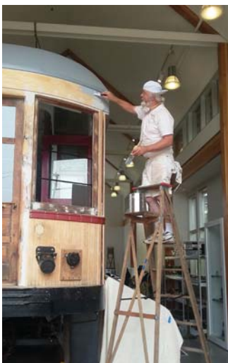
The tram car is primed and ready to paint.
