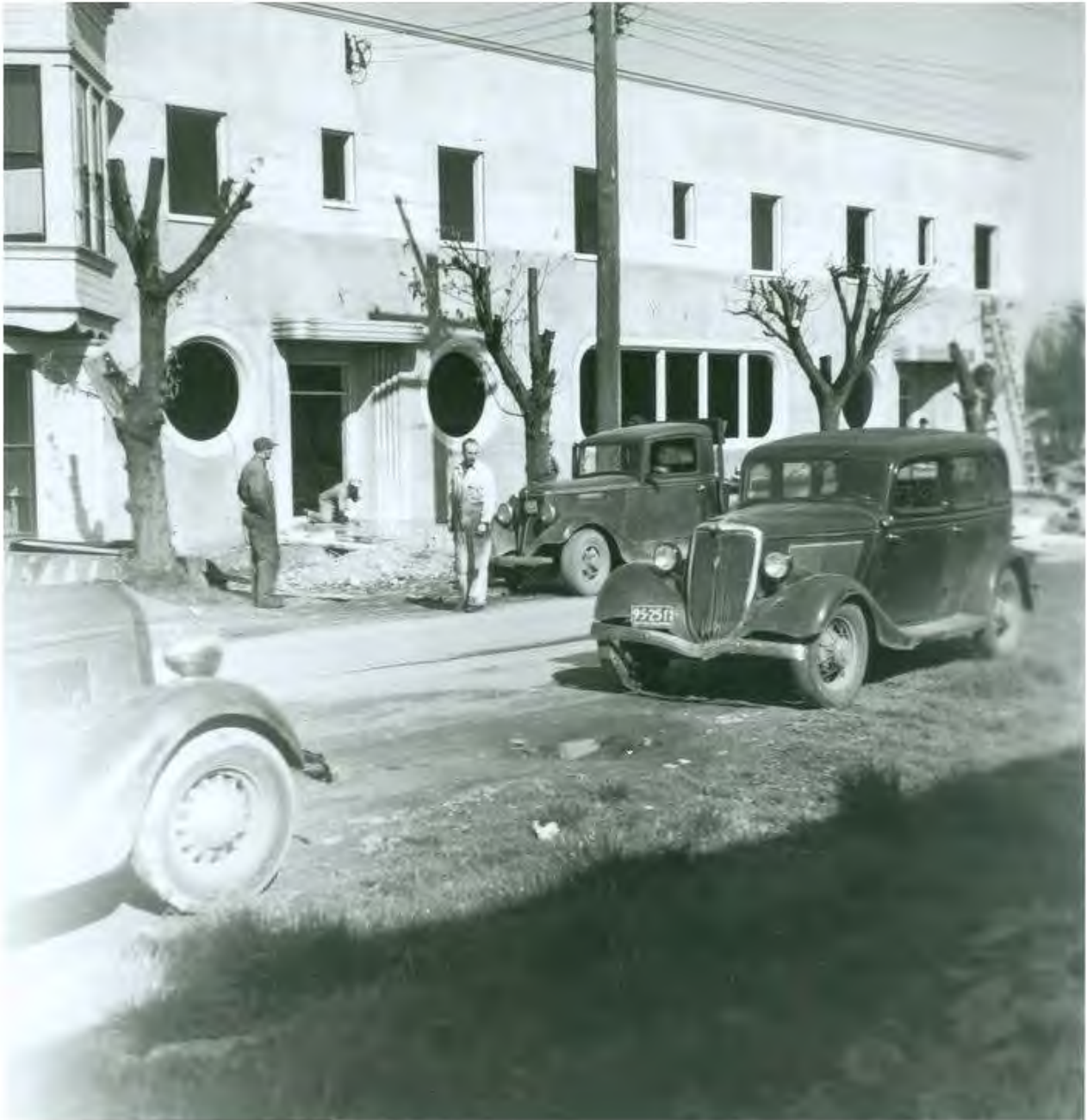
Steveston Hotel addition under construction, 1948 City of Richmond Archives, Photograph 1986 58 3.
