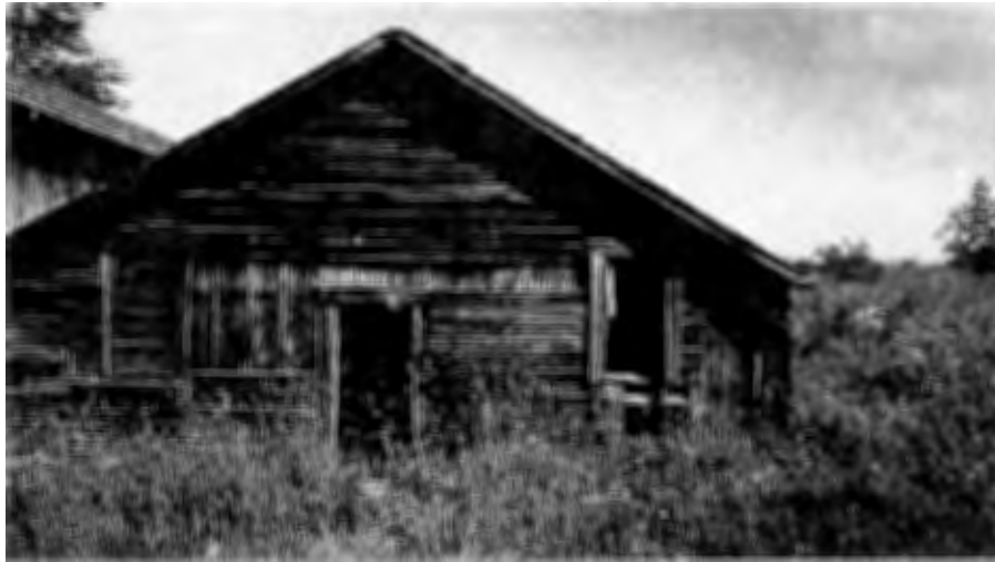
Murakami home in state of disrepair, before restoration, 1984, CRA 1984-4-56
