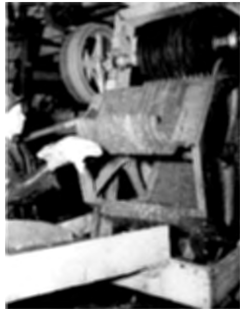
Worker using an "Iron Chink" to clean salmon, 1941, CVA 586-701
