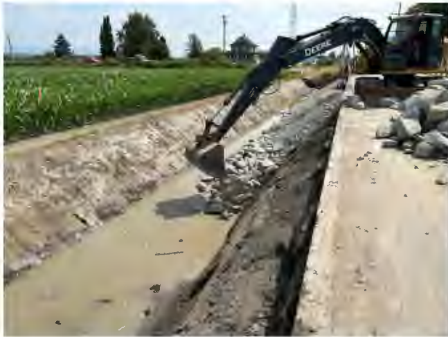
Canal Stabilization Works
