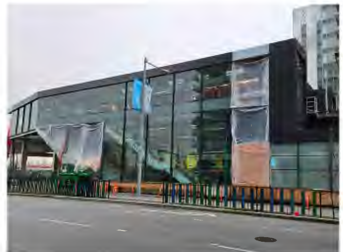
Capstan Station Construction
