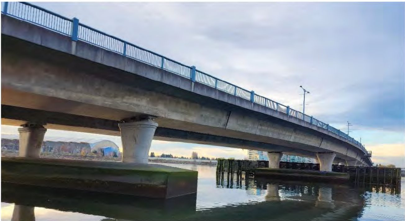
Bridge Condition Assessment
