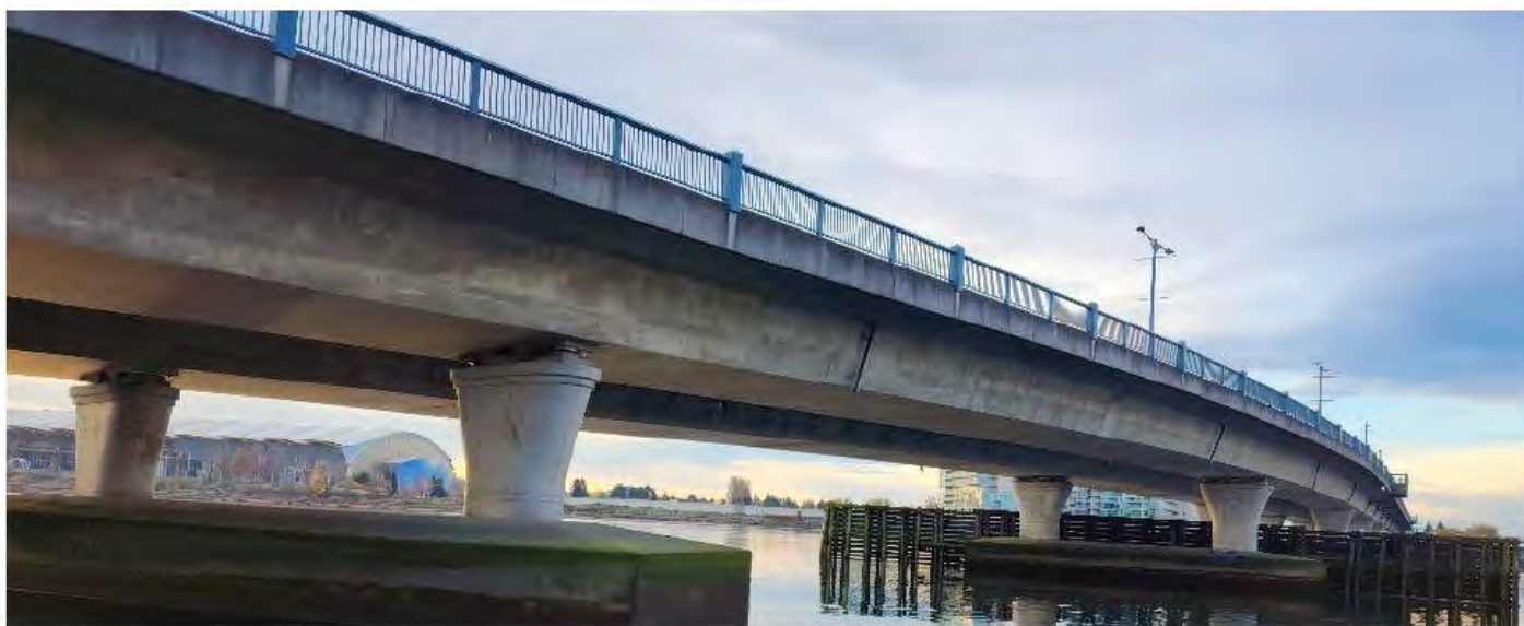
Bridge Condition Assessment
