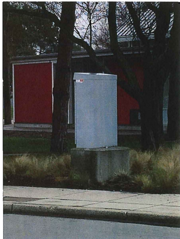
No. 1 Rd (Steveston Tram)
