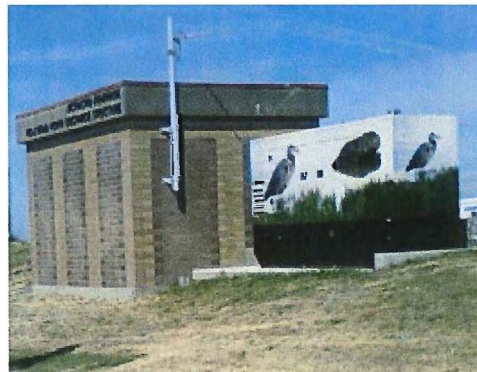
No 2 Rd Pump Station
