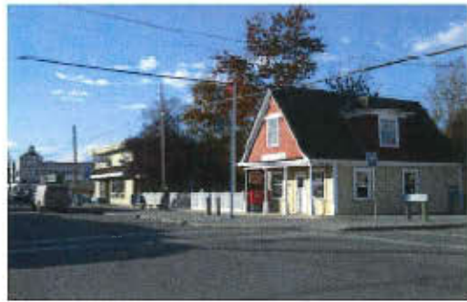
Moncton Street looking west
