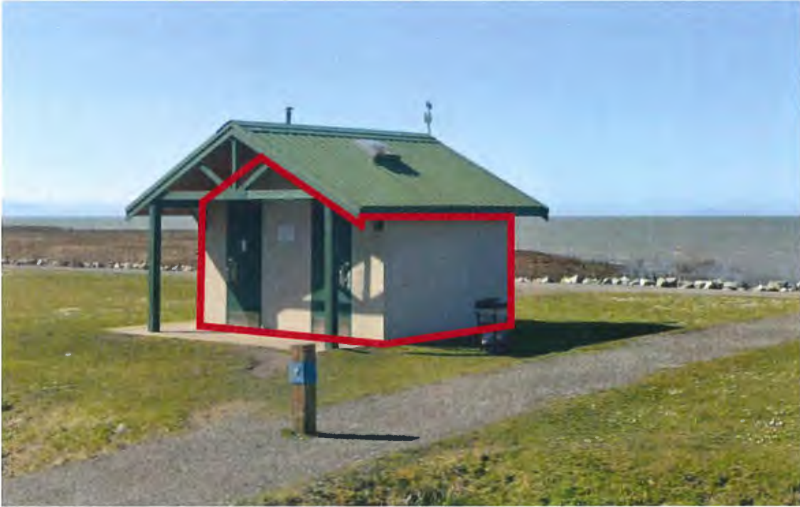
Proposed mural on Trail Washroom at Terra Nova Park (approx. 400 square feet)
