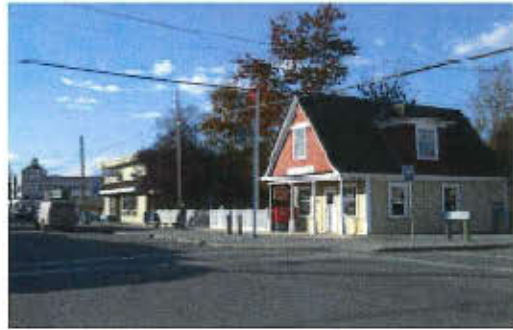
Moncton Street looking west
