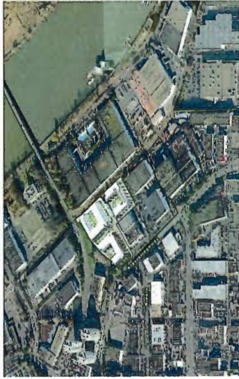
5 Site Aso View - Before
