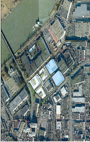
6 Site Aerial View
