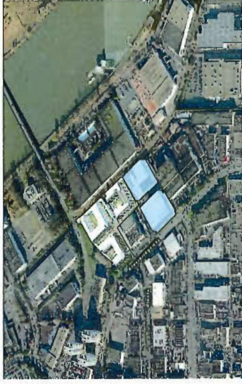
6 Site Aso View - After
