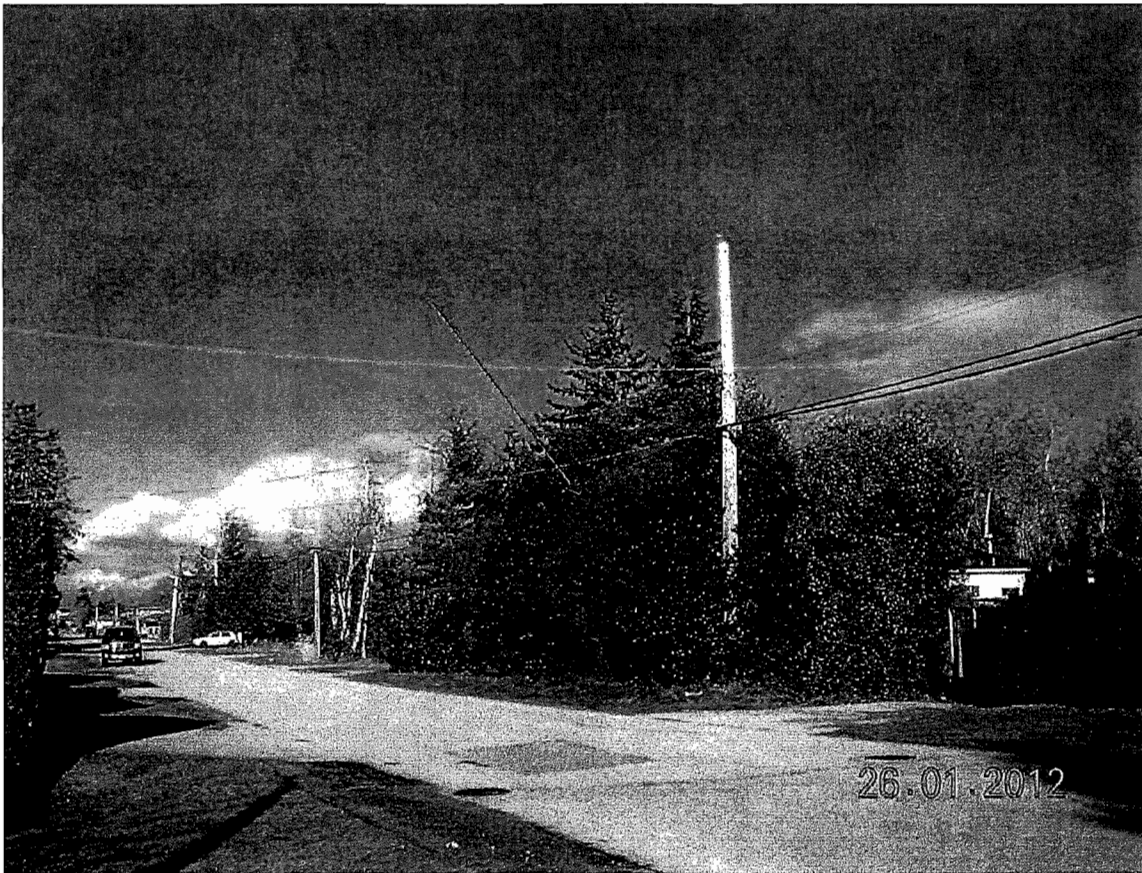
Photograph 1: Shows a hedgerow of off-site trees proposed for removal. These trees are located in the roadway easement adjacent to 7040 and 7060 Bridge Street. The development requires the permission from City of Richmond Parks Department to authorize the removal of the hedge.
