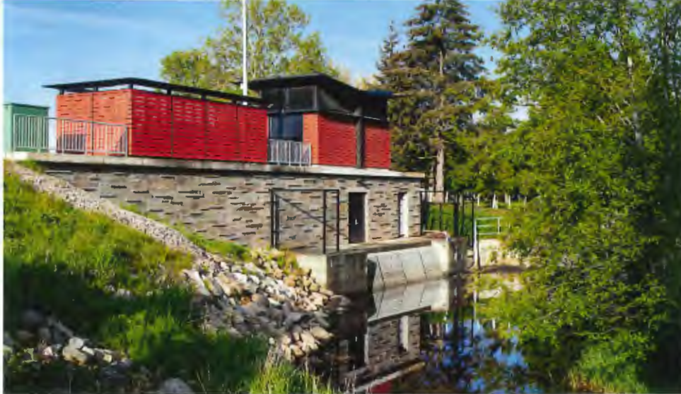
Figure 1. Horseshoe Slough Pump Station, City of Richmond
