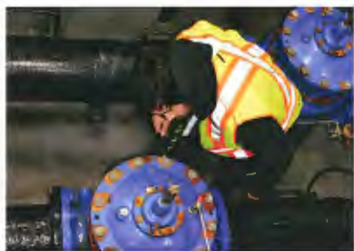
PRV station maintenance
