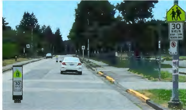
Figure 2: In-Street Marker on Fourth Avenue
