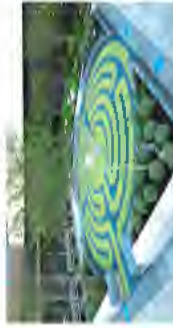
Street Bond Used for Marking Paving
