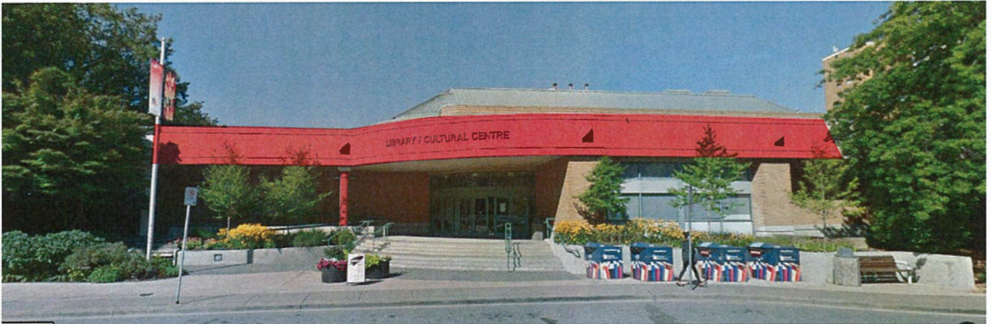
Figure 1 – Exterior fascia banding and columns, highlighted in red at Minoru Gate entrance.
