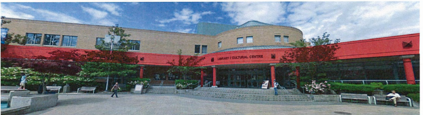
Figure 2 – Exterior fascia banding and columns, highlighted in red at Cultural Centre Plaza entrance.
