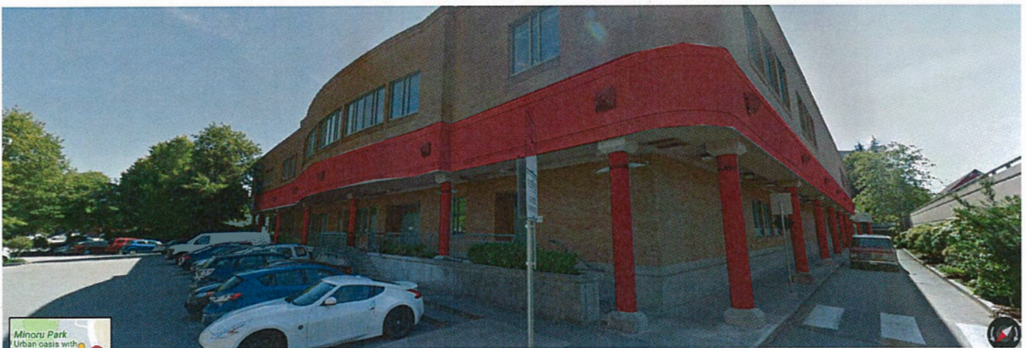
Figure 3 – Exterior fascia banding and columns, highlighted in red at north parking lot and east access lane.
