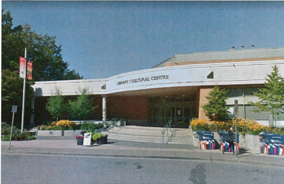
Figure 1. Richmond Cultural Centre, 7700 Minoru Gate.
