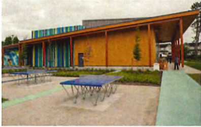
Amenities surrounding the energy centre at Alexandra Park.
