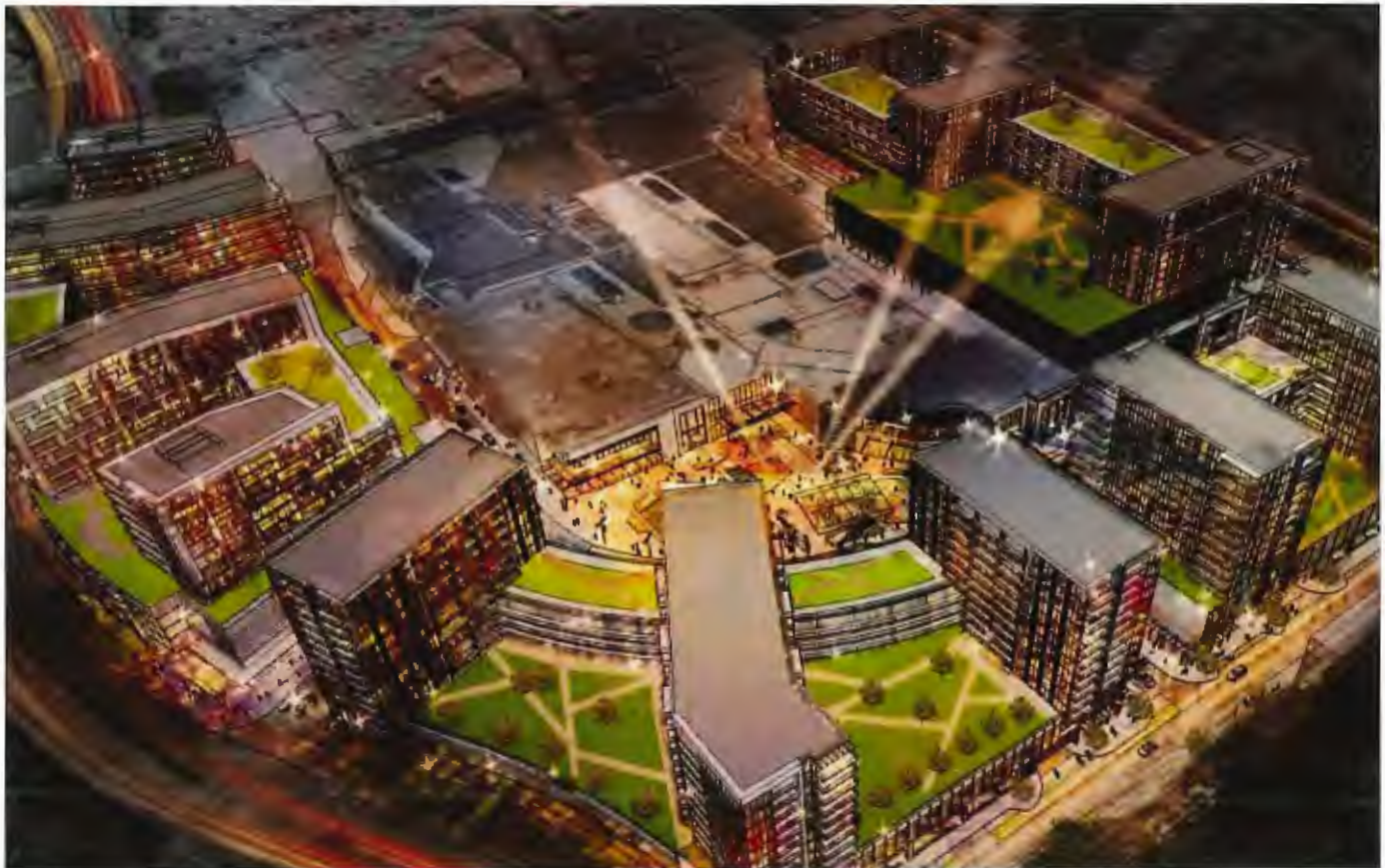
The Richmond Centre development currently under construction.
