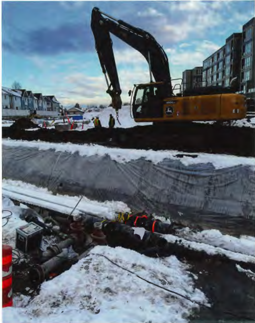
Implementing distribution piping in the ADEU.
