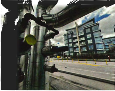
Riva 3, a building serviced in the OVDEU.
