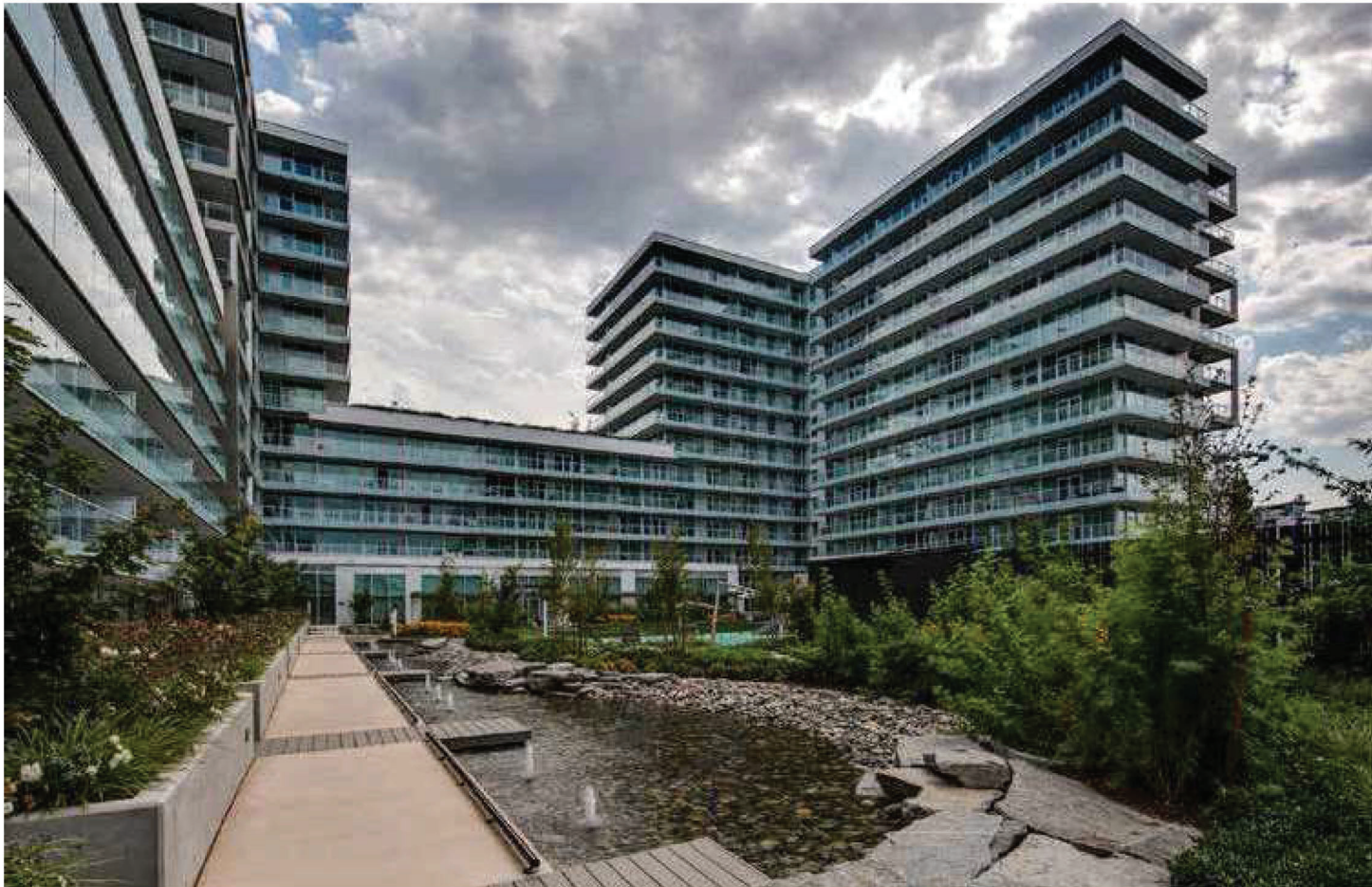
The number of district energy serviced buildings in Richmond continue to grow. The Paramount located at 6340 No. 3 Road.
