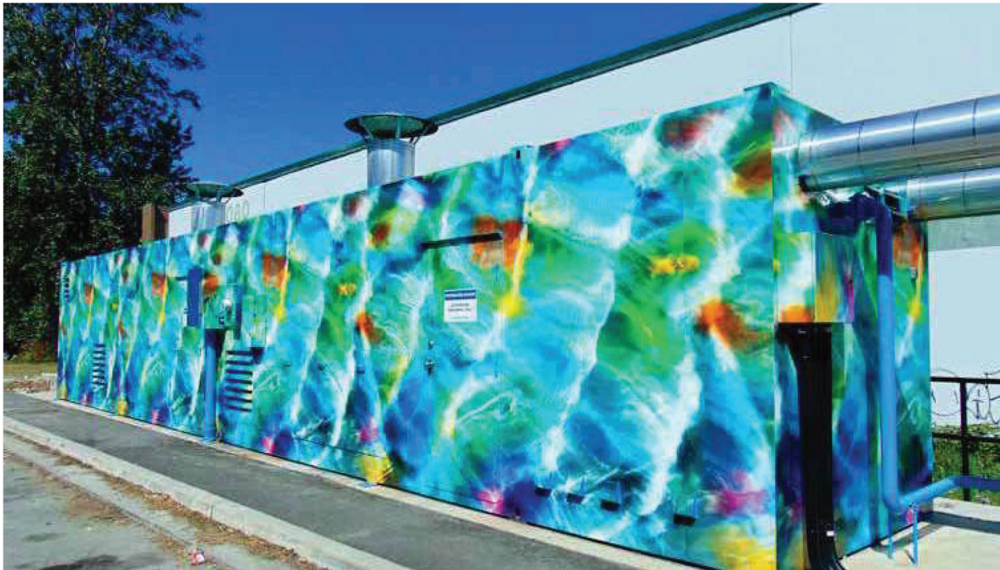
Oval Village’s interim energy centre
