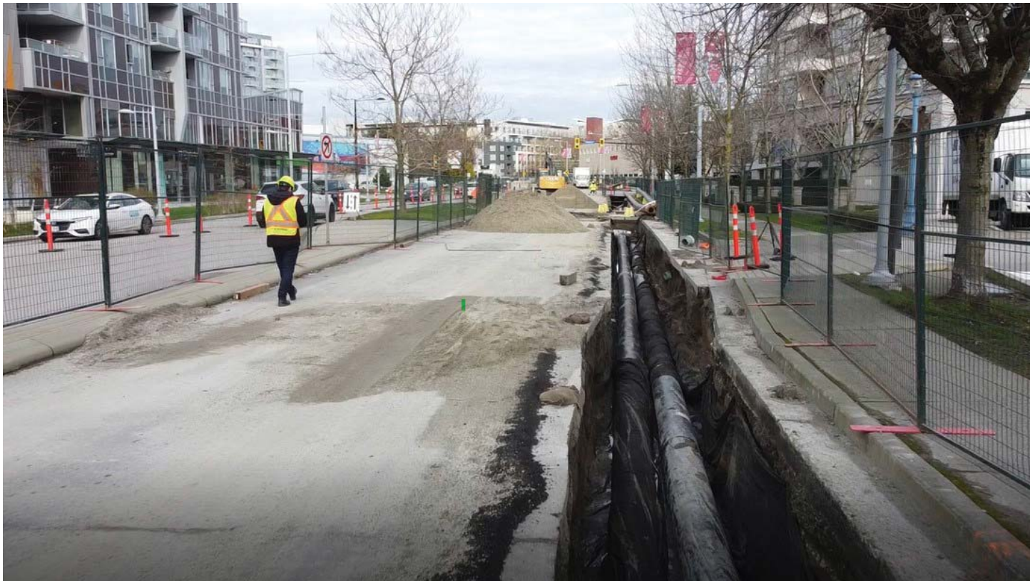
DPS piping is constructed along Gilbert Rd
