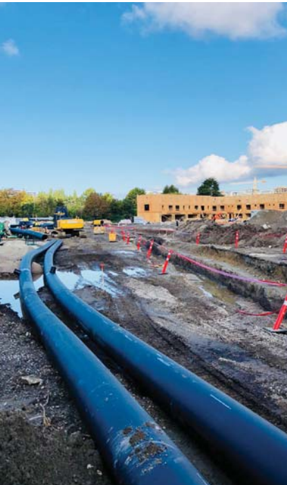
Distribution piping is staged in advance of construction at the ADEU
