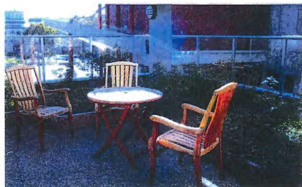
Barrier railings for a rooftop patio (Victoria, BC)
