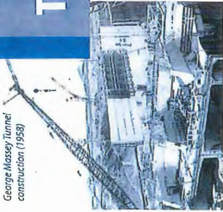
Sections of the Tunnel prior to placement under the river (1957)
