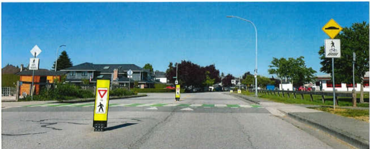
Figure 1: In-Street Pedestrian Zone Markers on Railway Avenue
