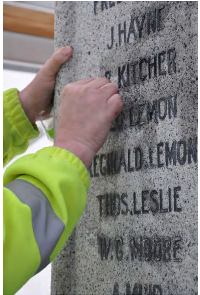
Legion Volunteer removes paint from the Cenotaph using acetone.
