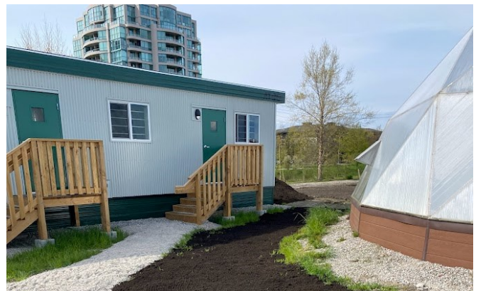
Farm office constructed on site Feb. 2022.
