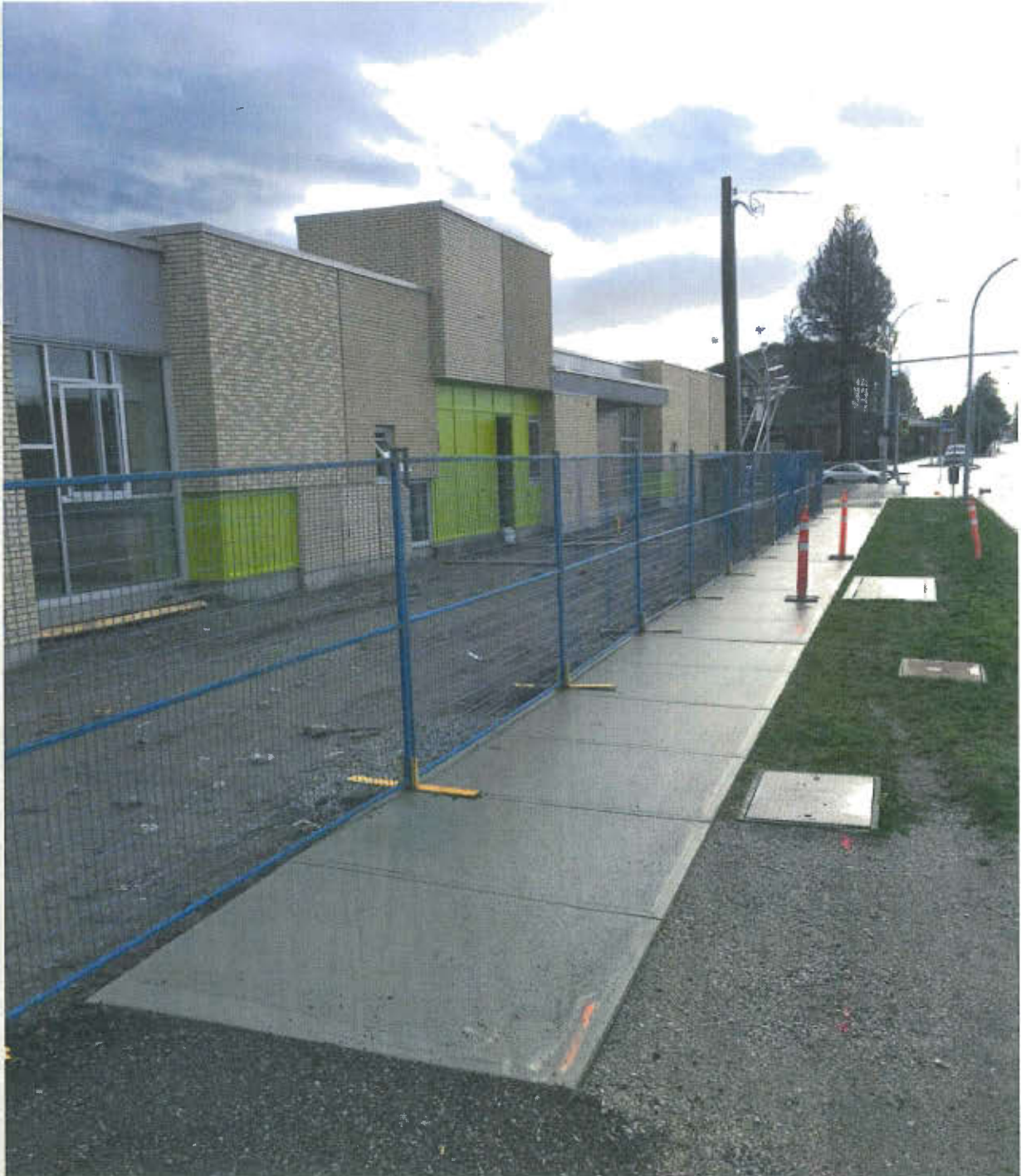
Photo of Building Under Construction
