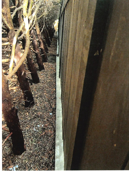
Photo 2 Existing CIP retaining wall along east property line
