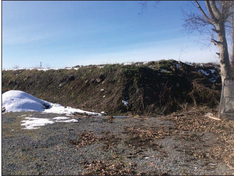
PHOTO 2. APPROXIMATELY 2.5 M OF FILL HAS BEEN PREVIOUSLY PLACED
