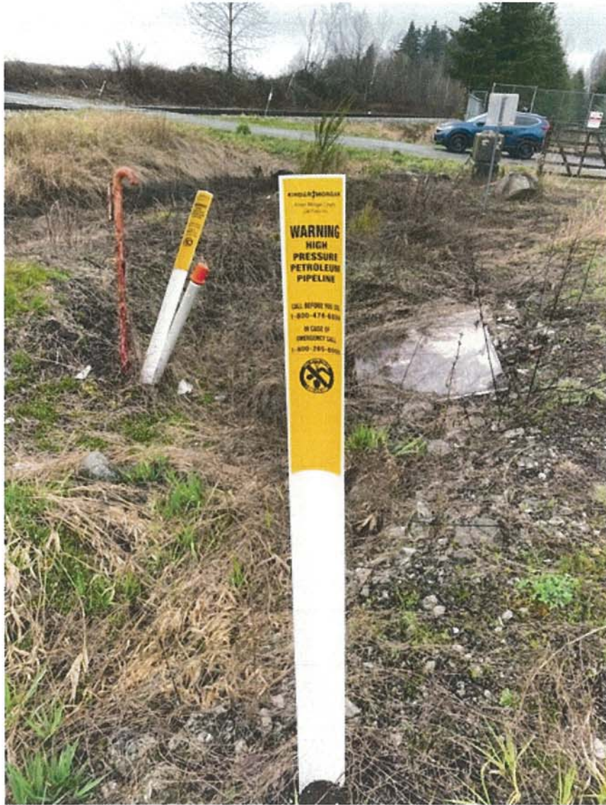
Figure 1 Kinder Morgan Pipeline ROW
