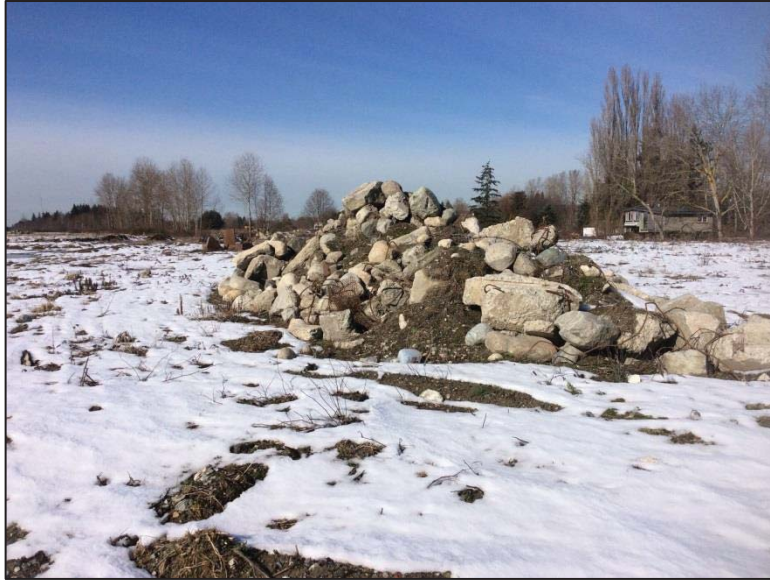
PHOTO 4. BOULDER, CONCRETE STOCKPILE SITUATED AT PM 7 IN THE PROPOSED PLACEMENT AREA.
