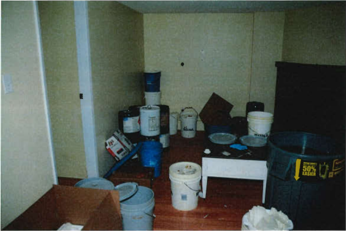
Image 1: various chemical drums found with unknown liquids in the downstairs living room.
