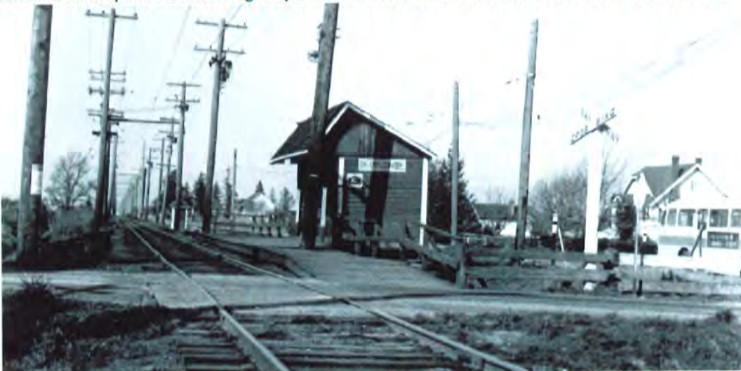
Branscombe Station ca. 1950, with subject house on the right. Source: City of Richmond Archives, Photograph #1978 21 30
