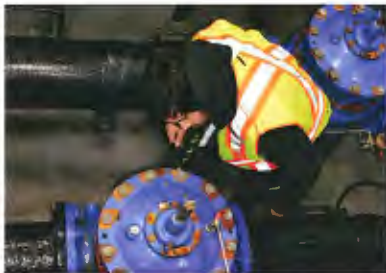
PRV station maintenance
