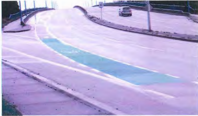
Figure 2: Green Surface in No. 2 Road Bike Lane
