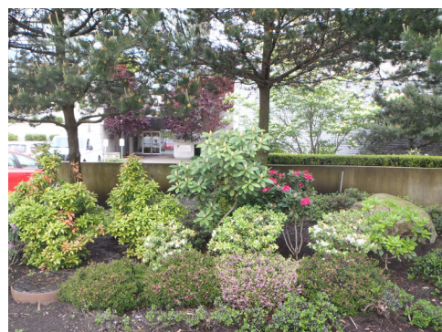
Implementation of rain gardens and rock trenches for detention on private properties.
