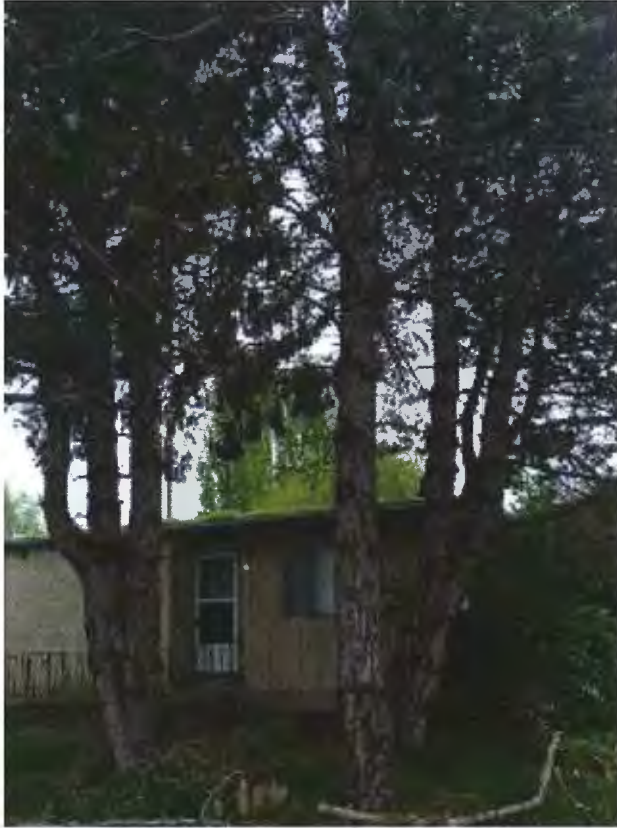
Figure 2 Pines to be removed for house demolition
