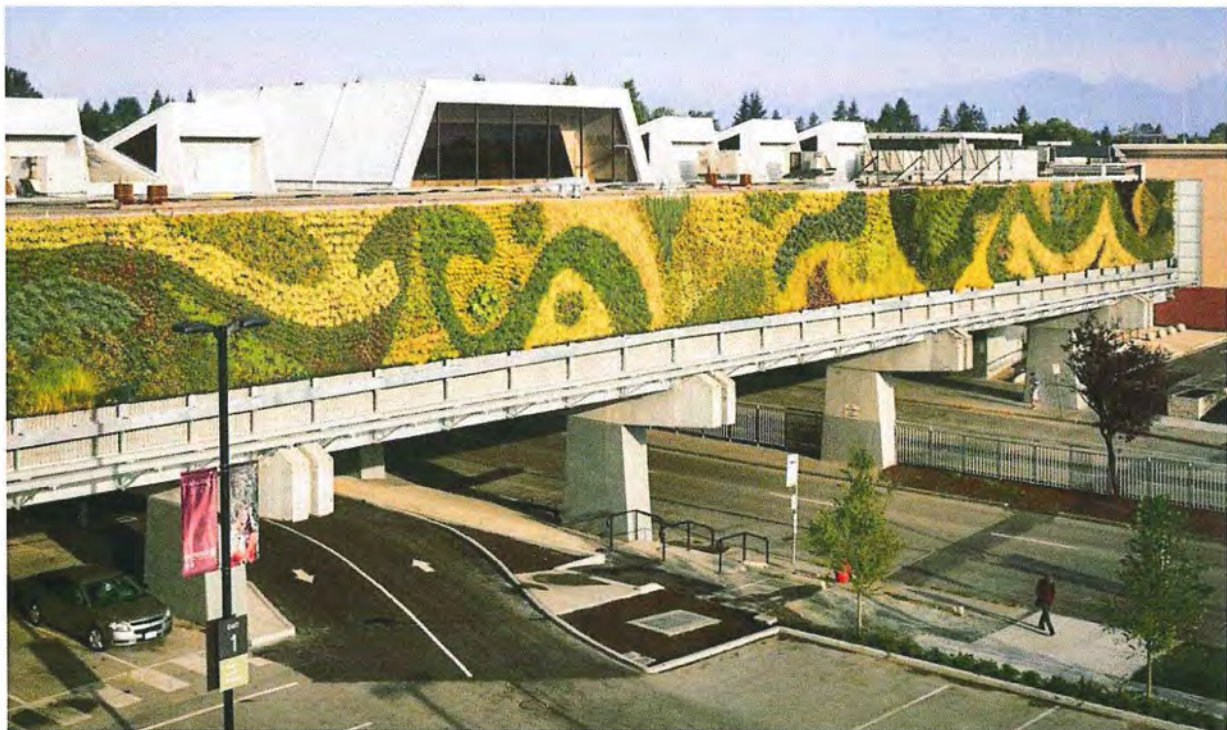
Green Wall at Guildford Town Centre [Source: Green Over Grey – Living Walls and Design Inc., Vancouver, BC]
