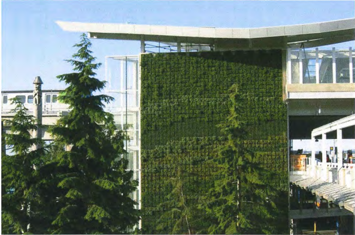
Green Wall at Vancouver International Airport [Source: Connect Landscape Architecture Inc., Vancouver, BC]
