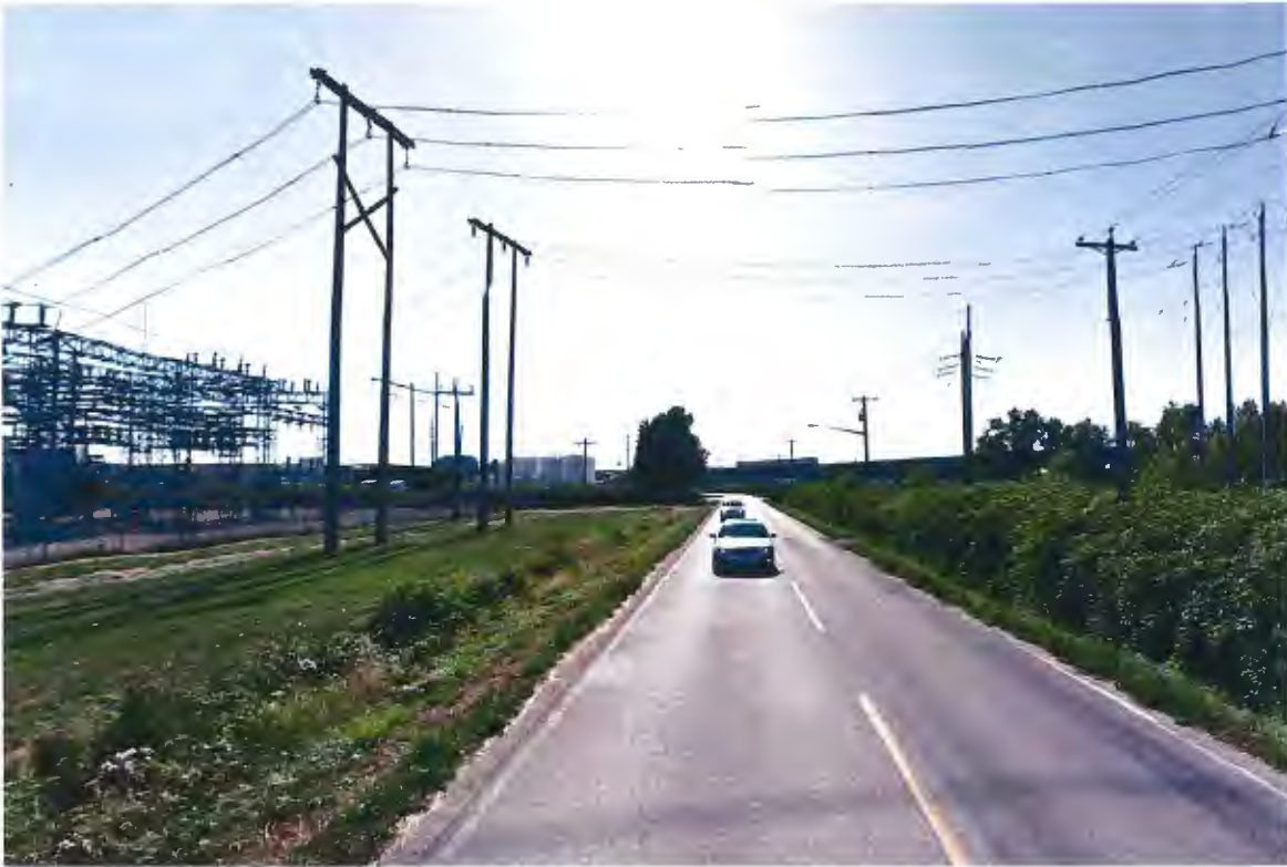
Before: Existing River Drive looking west (west of No. 4 Road)
