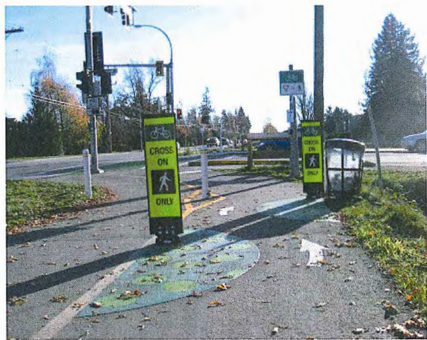
Figure 2: Railway Greenway Signage & Pavement Markings
