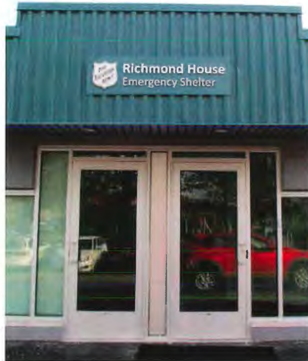
The new emergency shelter provides safe and secure shelter spaces in a supportive environment for up to 36 people—more than triple the number that existed previously.
