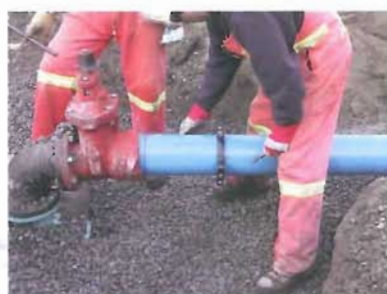
Installing a PVC pipe
