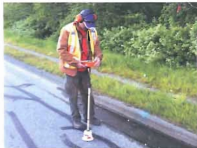
Using a logger for leak detection
