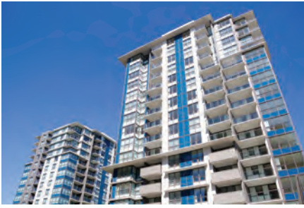
Kiwanis Towers, Richmond
