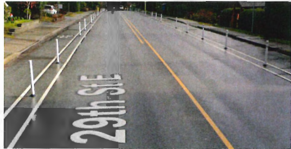
Figure 1: Example of Buffered Bike Lane with Delineator Posts (29 th St E, North Vancouver)
