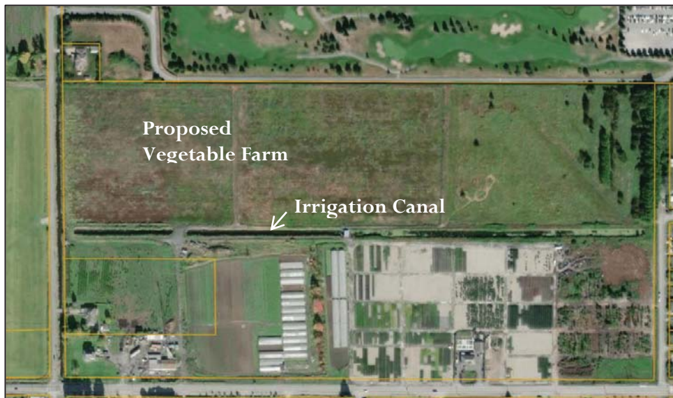
FIGURE 1. IRRIGATION CANAL SITUATED THROUGH THE CENTRE OF THE PROPERTY. OVERHEAD SPRINKLER SYSTEMS AND DRIP IRRIGATION CAN BE CONNECTED TO THIS. MAP IMAGERY FROM IMAPBC 4.0.
