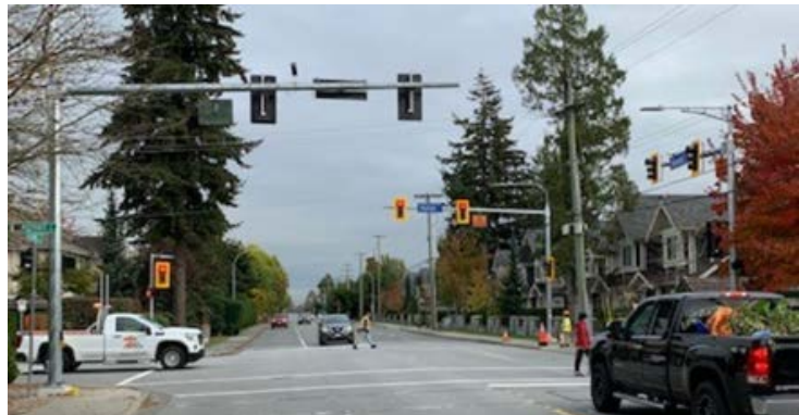
Figure 1: Upgrade of Pedestrian Signal at Blundell Road-Moffat Road to Full Signal
