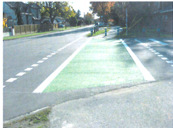
Figure 3: Enhanced Crosswalk on Saunders Road at Garden City Road
