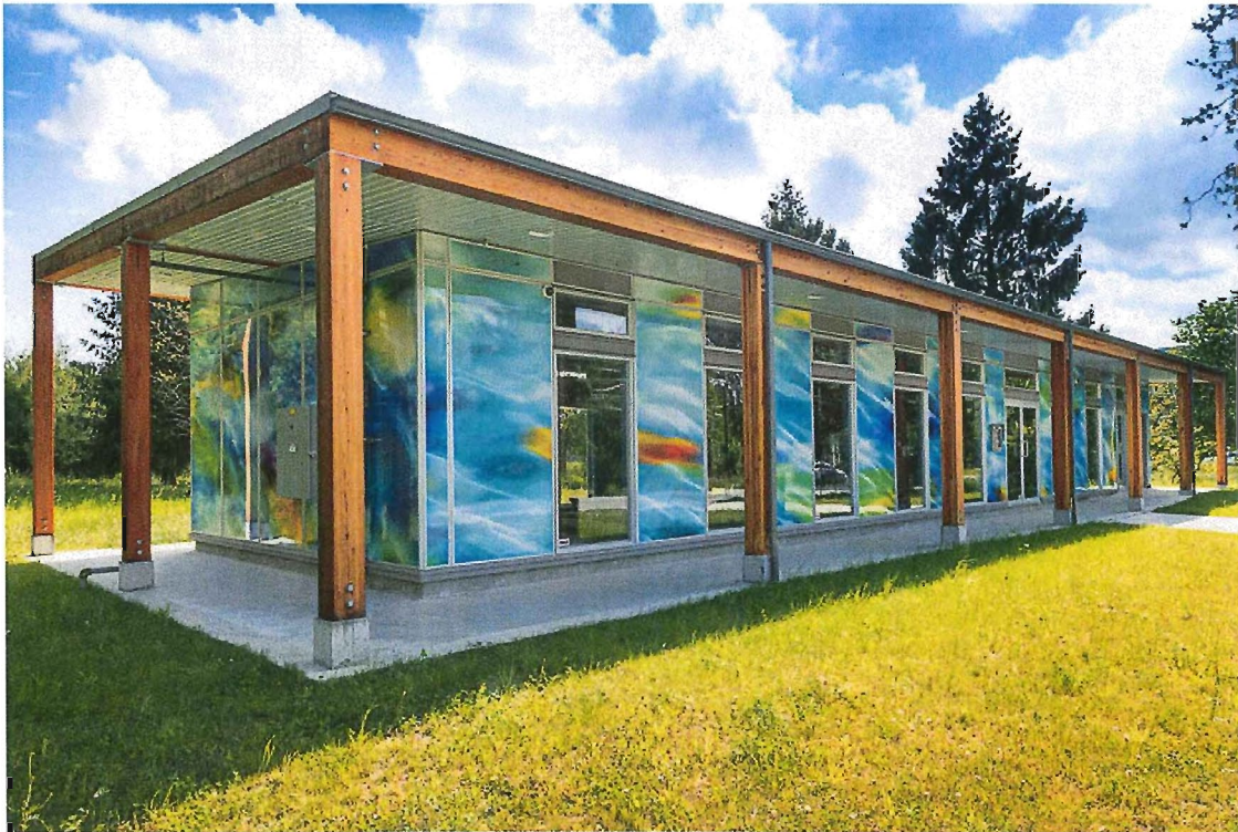
Current , Andrea Sirois, 2012. City of Richmond Alexandra District Energy Utility Building
