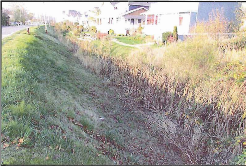
Photograph 3. West view of frontage ditch; adjacent property has pedestrian pathway, manicured lawn and planted ornamental species within and adjacent to the ditch (November 05, 2012).
