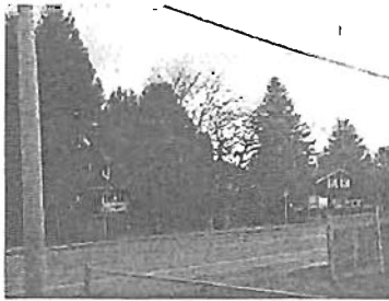
Low overhead wiring at site
