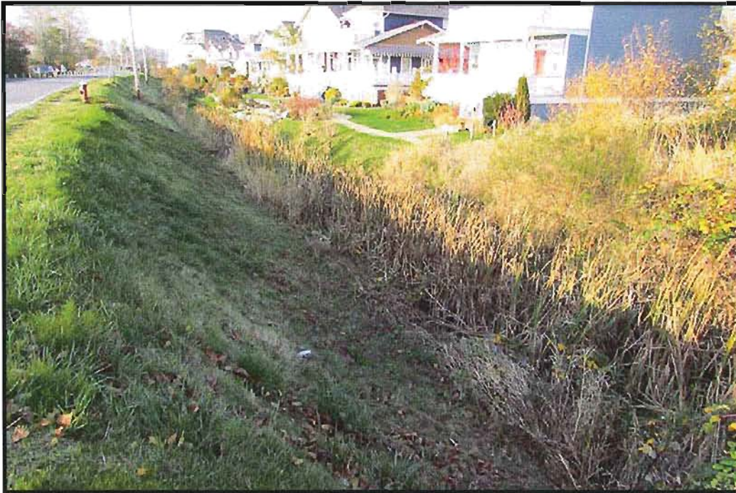
Photograph 3. West view of frontage ditch; adjacent property has pedestrian pathway, manicured lawn and planted ornamental species within and adjacent to the ditch (November 05, 2012).
