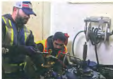
Pressure management system installation
