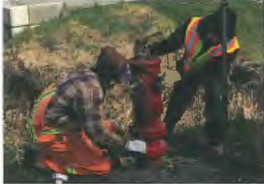
Servicing a fire hydrant
