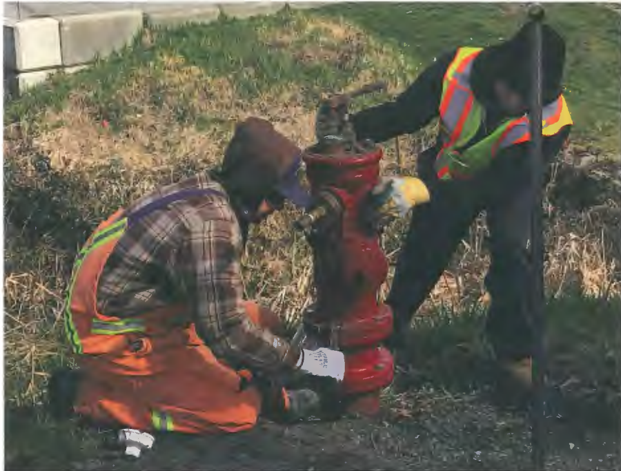
Servicing a fire hydrant
